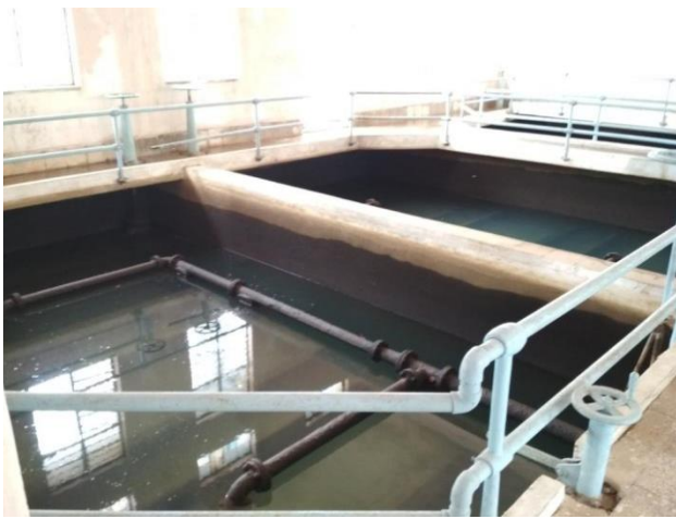
Filter Bed (Existing)
