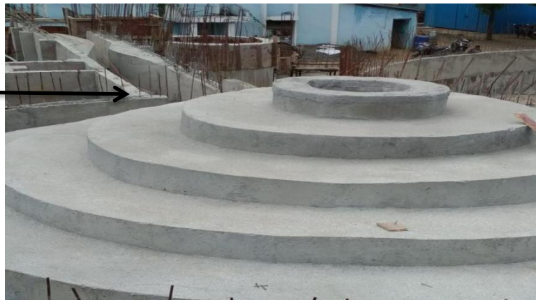
Figure 7. Parshall Flume
